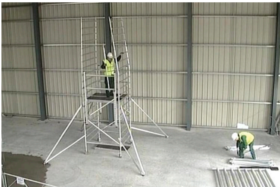
Figure 11 Advanced guard rails
