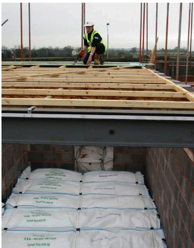
Figure 15 Soft landing system
