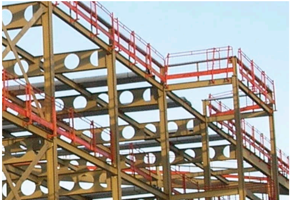
Figure 28 Edge protection installed with the steelwork
