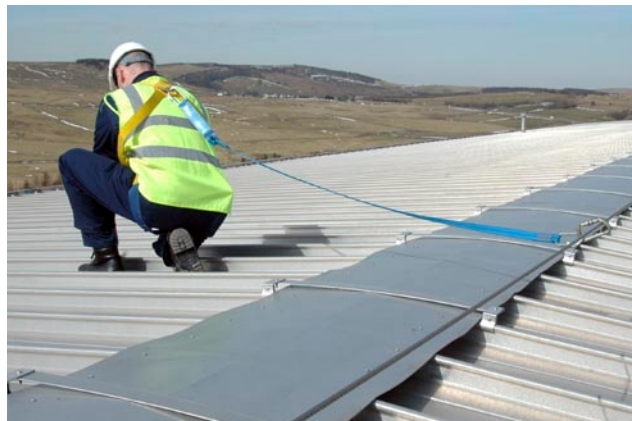
Figure 16 A work-restraint harness
