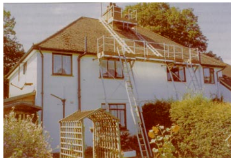
Figure 25 Proprietary access system for roof-work
