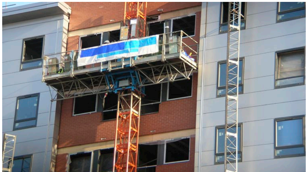
Figure 14 A mast climbing work platform
