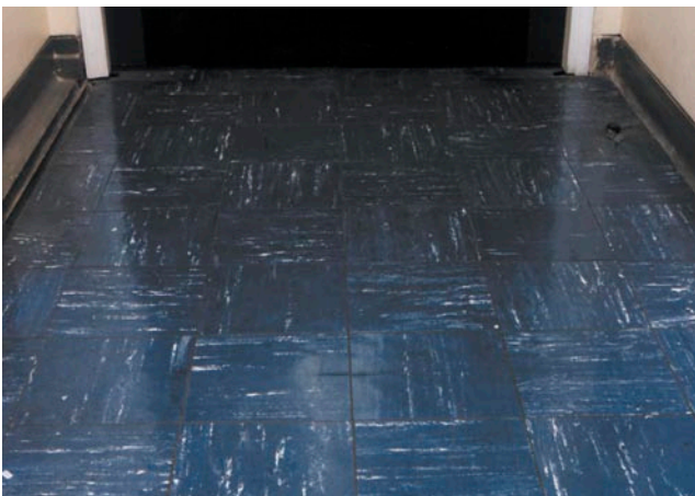
Figure 48e Asbestos-containing vinyl floor tiles
