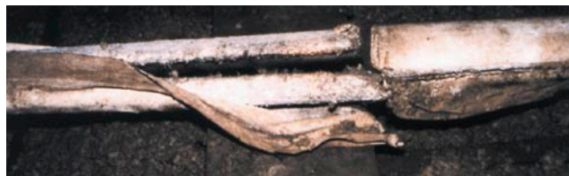
Figure 48a Asbestos-insulated water pipes showing evidence of maintenance work damage, with detached preformed sections and calico wrapping
