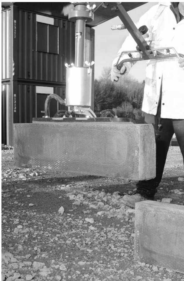
Figure 38 Handling kerbs using a vacuum lifter
